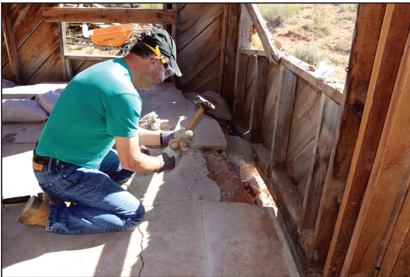
Co-Op member Richard Walker removes unsupported concrete flooring.
