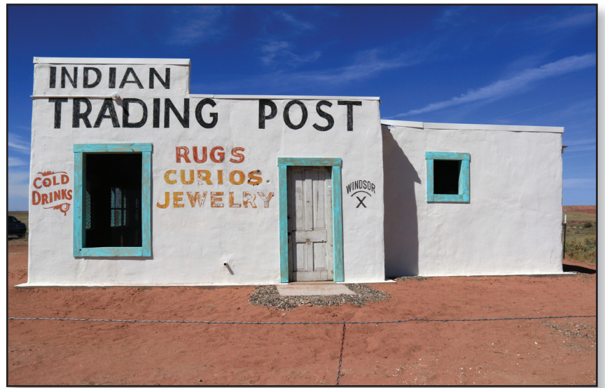
The completed east wall of the trading post.
