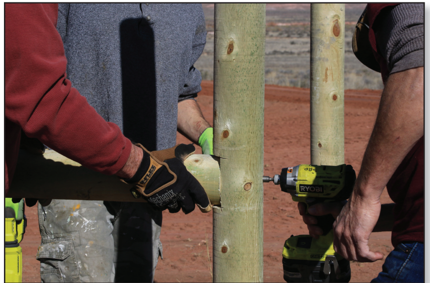
Crew members assemble corner posts.
