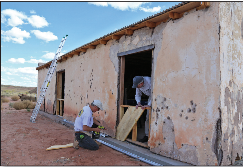
Sheathing is replaced under the rear windows.
