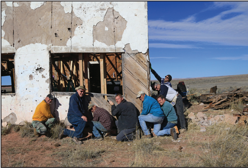
A humorous attempt at lifting the southeast corner.
