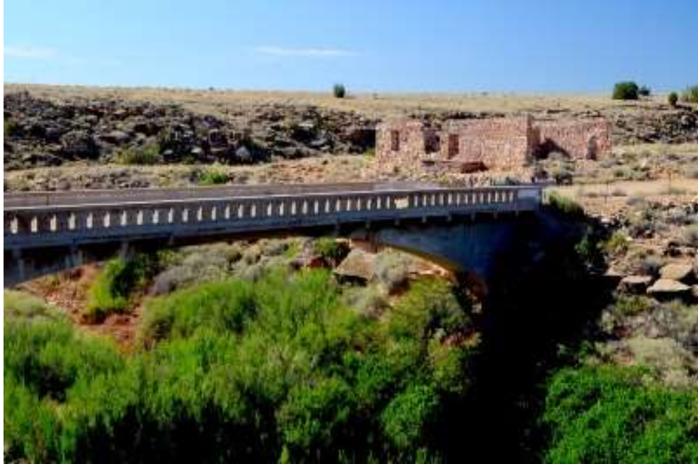
The bridge as seen from the store with the 2 nd zoo on the left.
