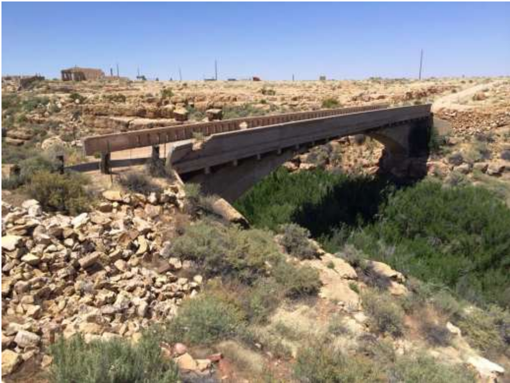
The bridge as seen from the Ticket Office (3.3)
